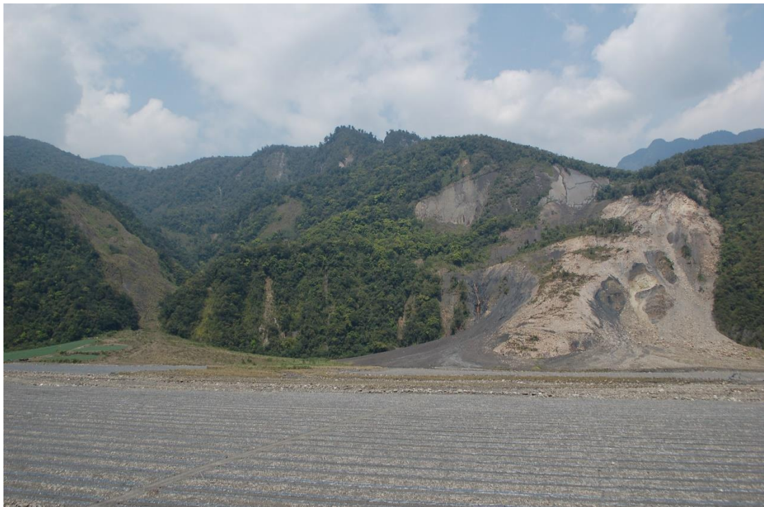
Figure 15. A landslide complex next to Cilan Mountain Cypress Forest on the main stream of Langyang River.
