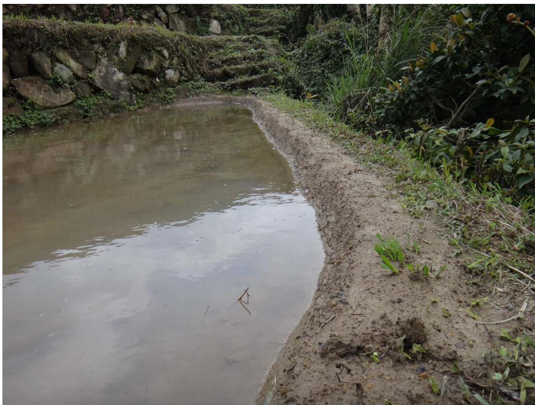
(b)田埂邊坡維護後樣貌
